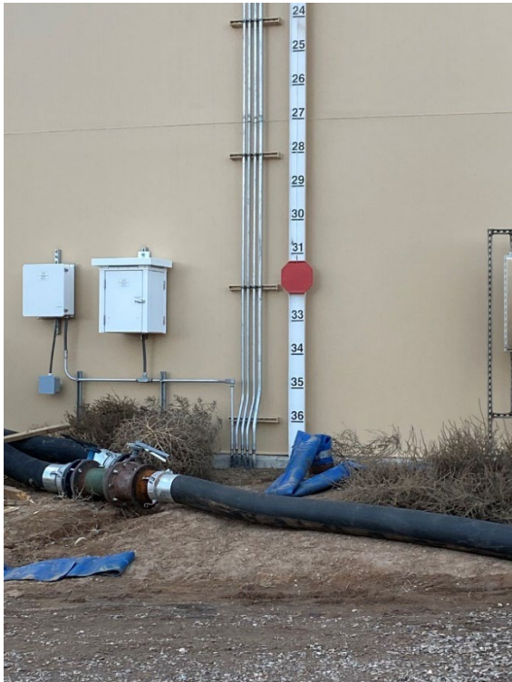
Filling storage tank.
