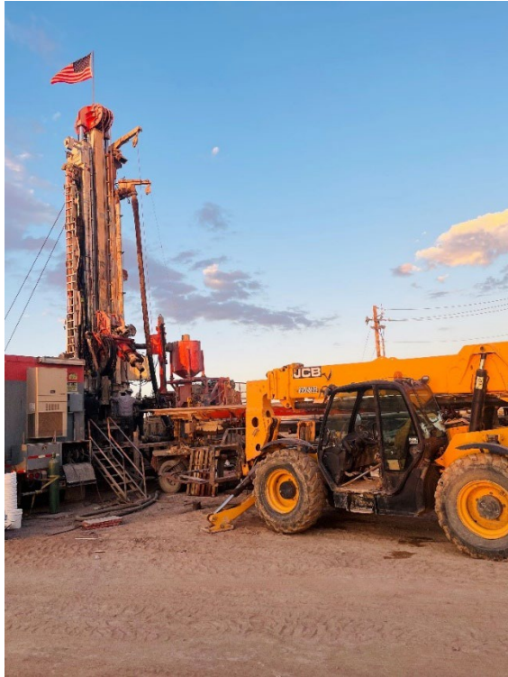
Running pipe for zone development.
