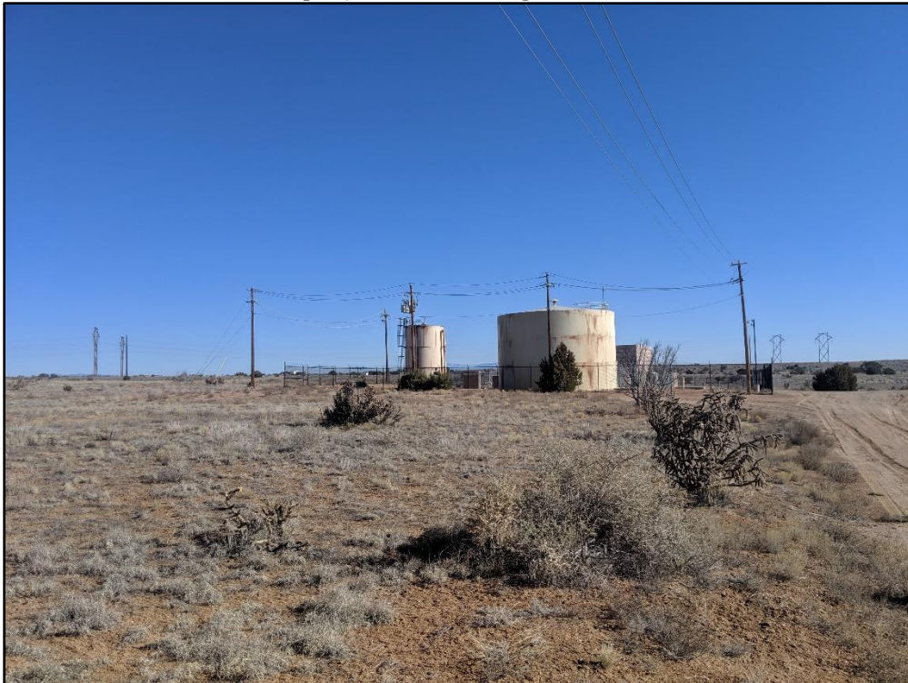
Photo 2. From southern project area facing north.
