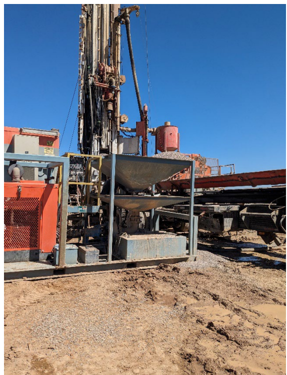
Gravel packing for zone sampling.
