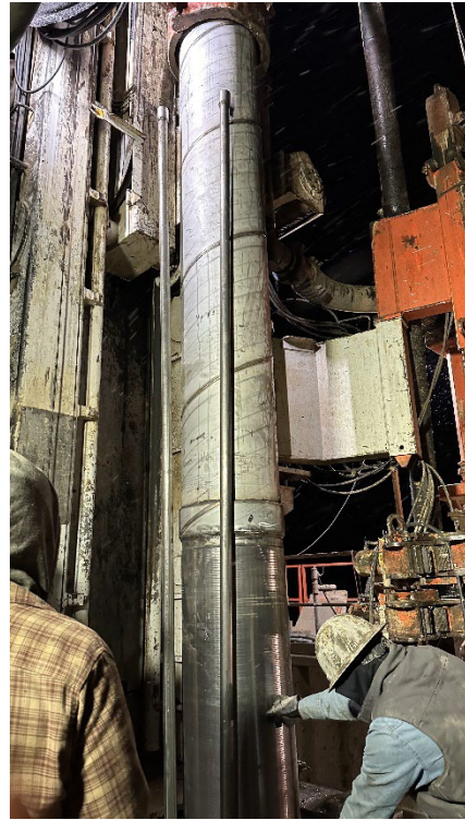
Running in casing and sounding tube.
