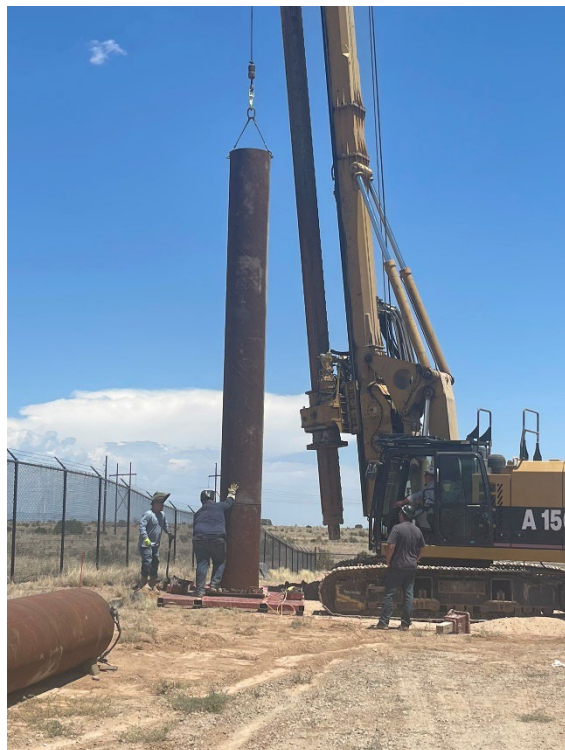
Running conductor casing.
