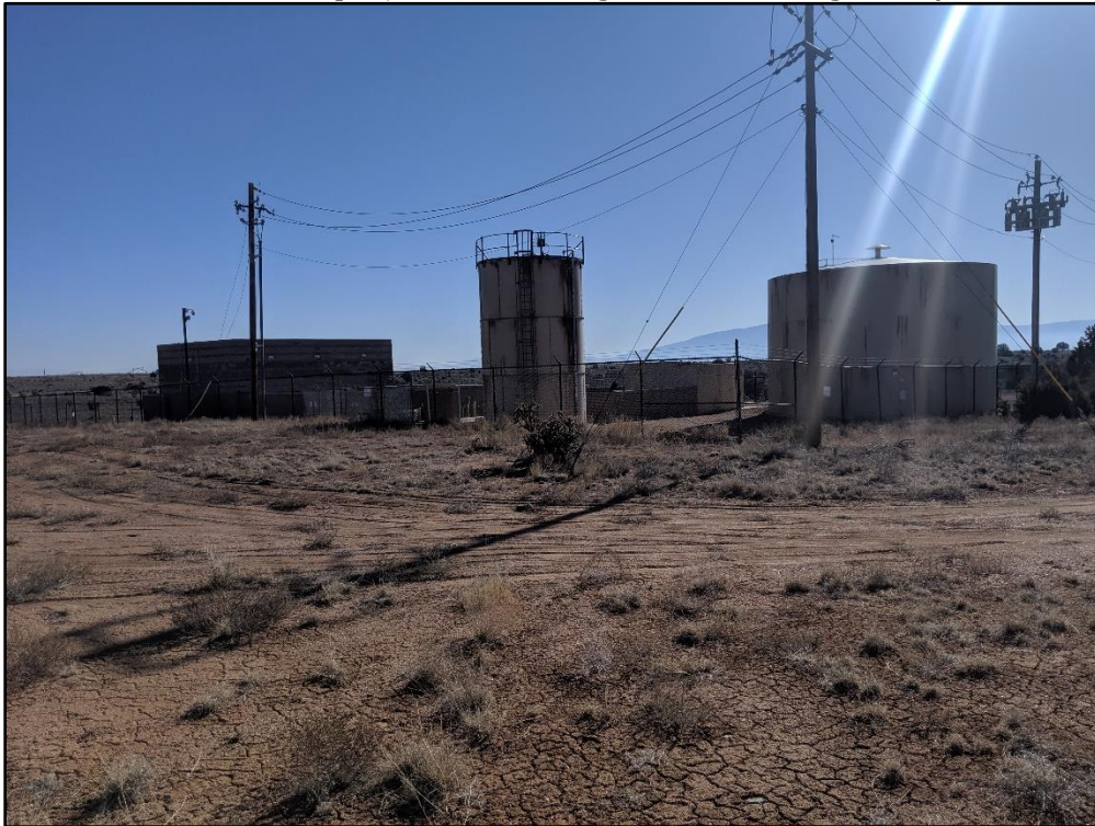
Photo 4. From central project area facing east to existing facility.
