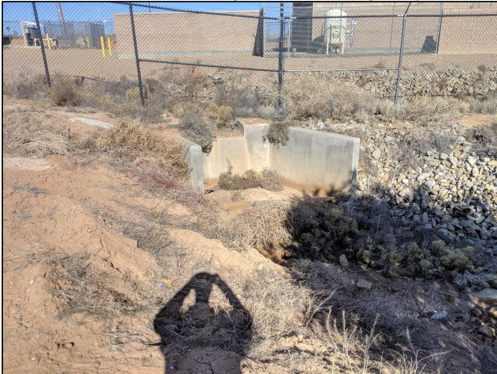
Photo 6. Outfall feature at eastern perimeter of existing facility.
