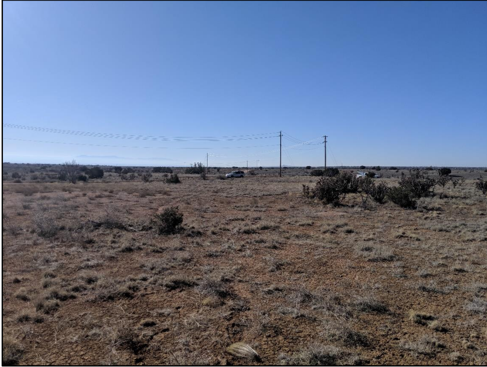
Photo 5. Facing southeast to property that will be acquired from AMREP.
